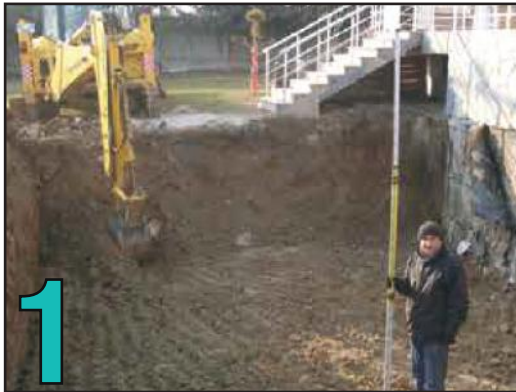
Excavation appropriate to pool design
