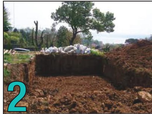
Excavation appropriate to pool design
