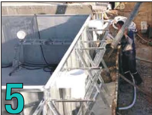
Concrete laying to supports
