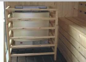
Wooden frame for protecting sauna heat generator
