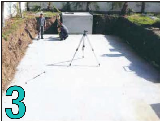
Substructural concrete laying
